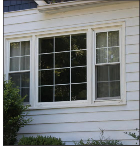
Figure 8.5. 121 Pisgah Drive, Window Detail, West Side
