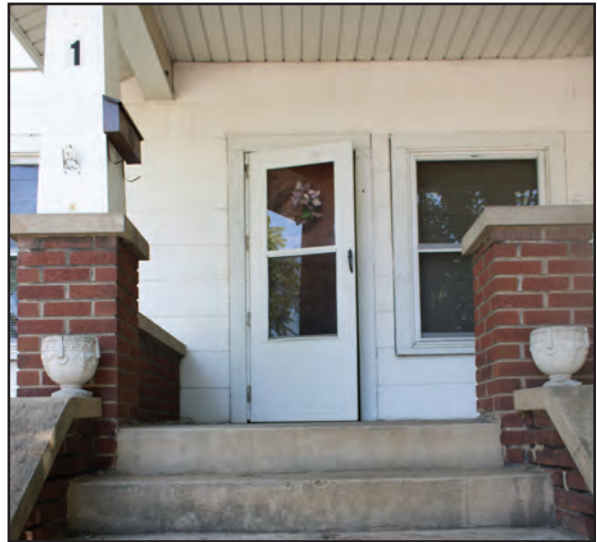
Figure 4.7. 1 Holtzclaw Street, Front Door Detail
