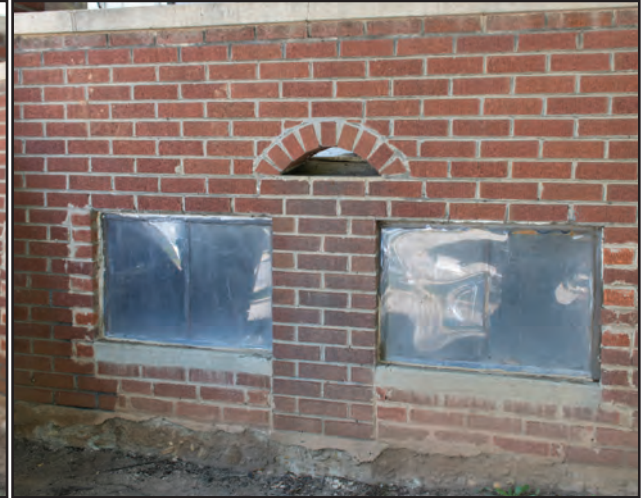
Figure 4.10. 1 Holtzclaw Street, Detail of Porch Vent and Basement/Crawl Space Windows
