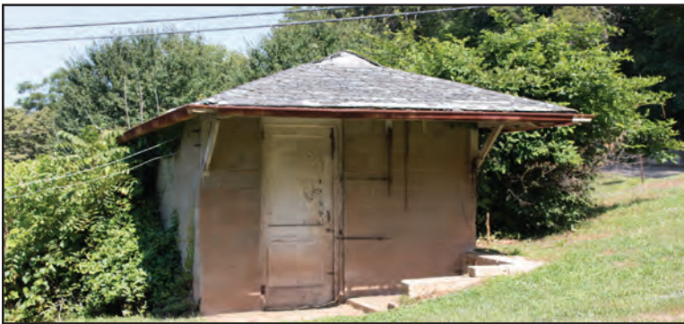
Figure 4.16. 1 Holtzclaw Street, Shed, East Side
