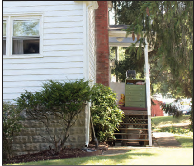
Figure 8.8. 121 Pisgah Drive, Rear Porch
