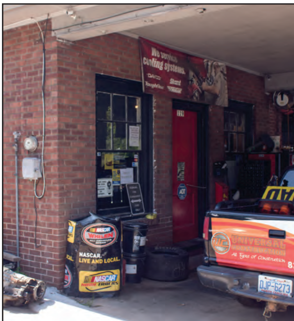
Figure 3.6. Howard Amoco, Canopy and Office
