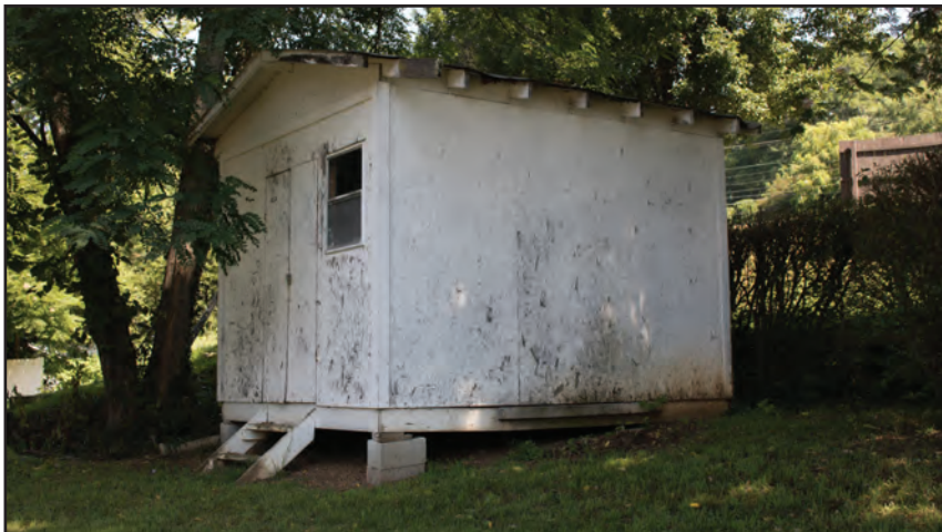
Figure 7.13. 120 Pisgah Drive, Shed
