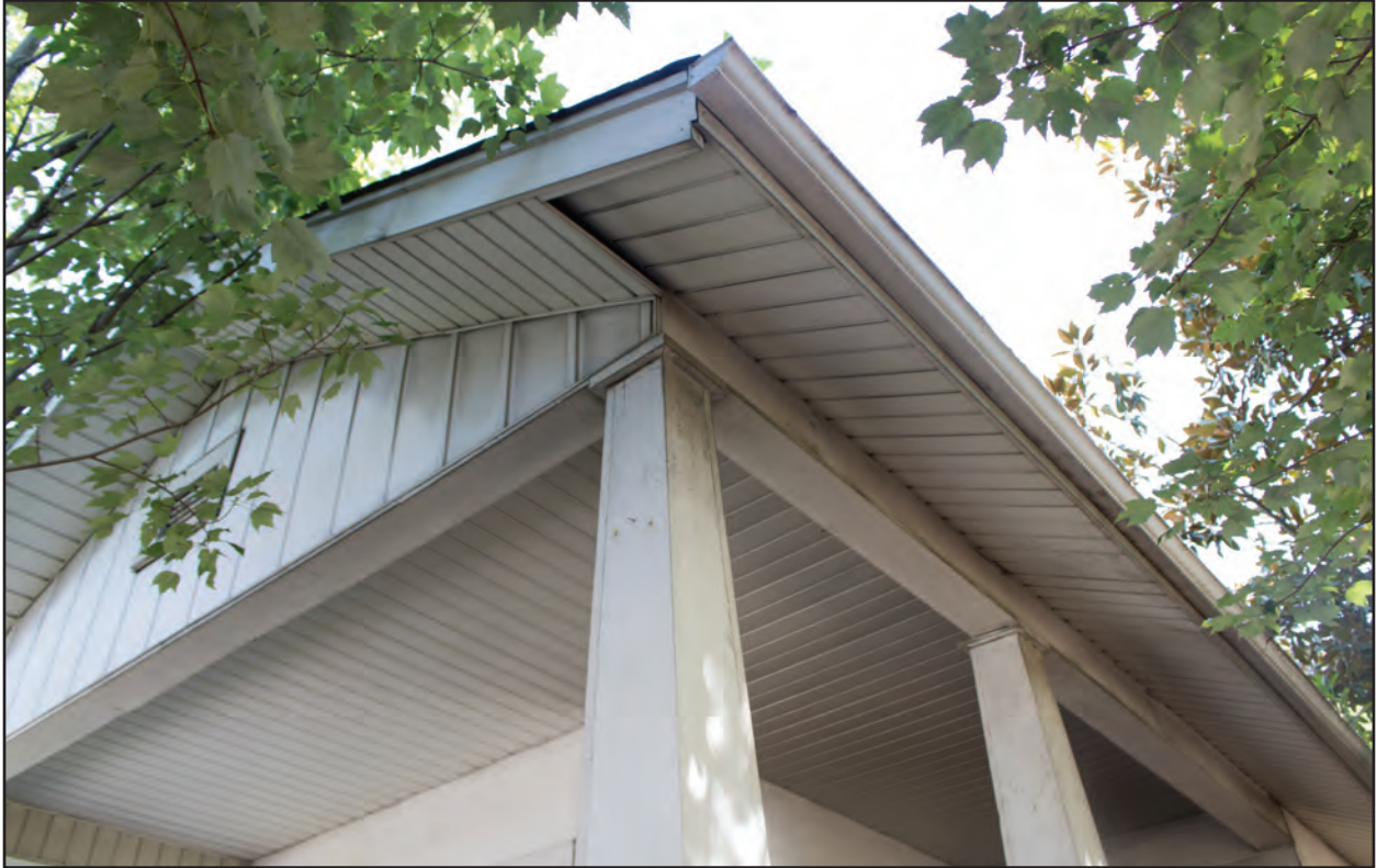
Figure 4.4. 1 Holtzclaw Street, Eave Detail
