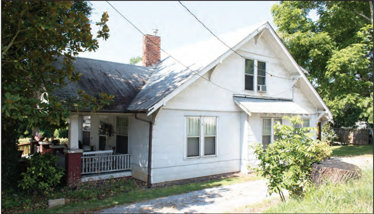
Figure 7.7. 120 Pisgah Drive, North Side
