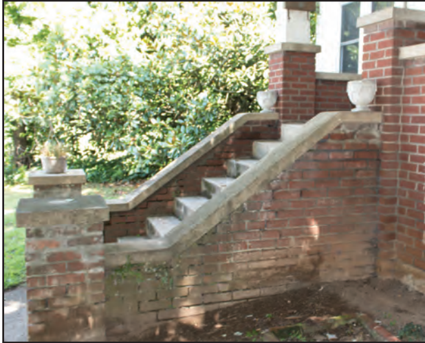
Figure 4.9. 1 Holtzclaw Street, Detail of Porch Steps
