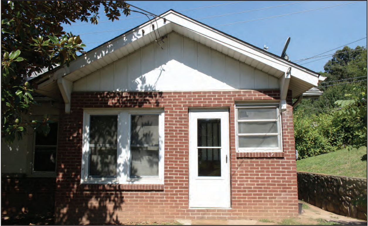
Figure 4.12. 1 Holtzclaw Street, East Side
