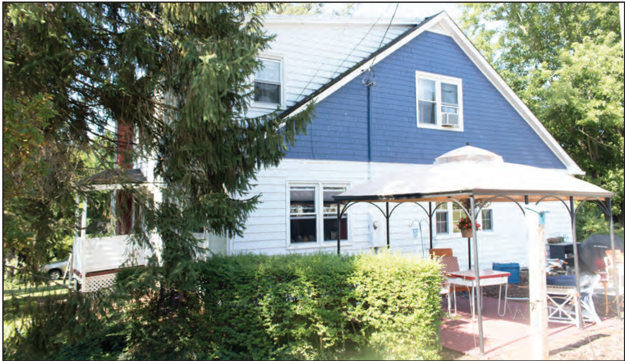
Figure 8.9. East and North Sides Oblique
