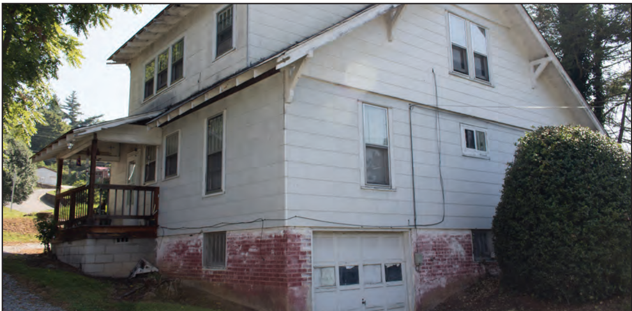
Figure 7.11. Oblique of West and South Sides
