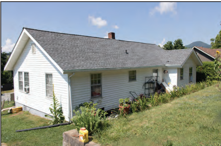
Figure 6.8. 115 Pisgah Drive, East and North Oblique
