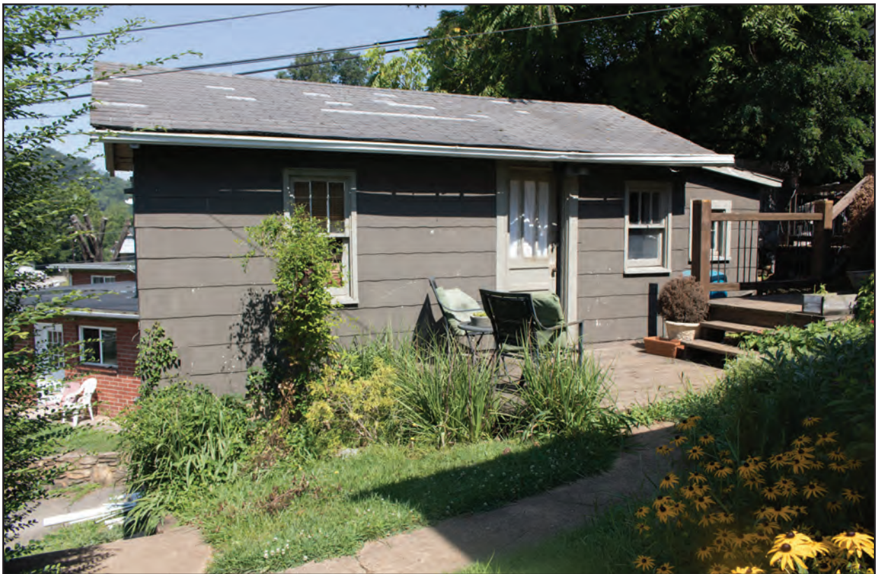
Figure 5.13. Garage, Upper Floor, East Side
