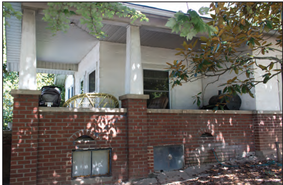
Figure 4.8. 1 Holtzclaw Street, East Side of Porch
