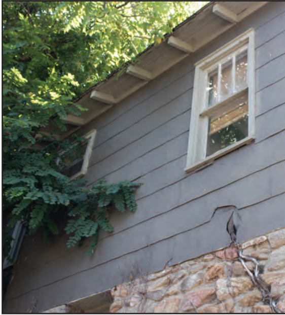
Figure 5.11. Garage, West Side, Siding and Window Detail
