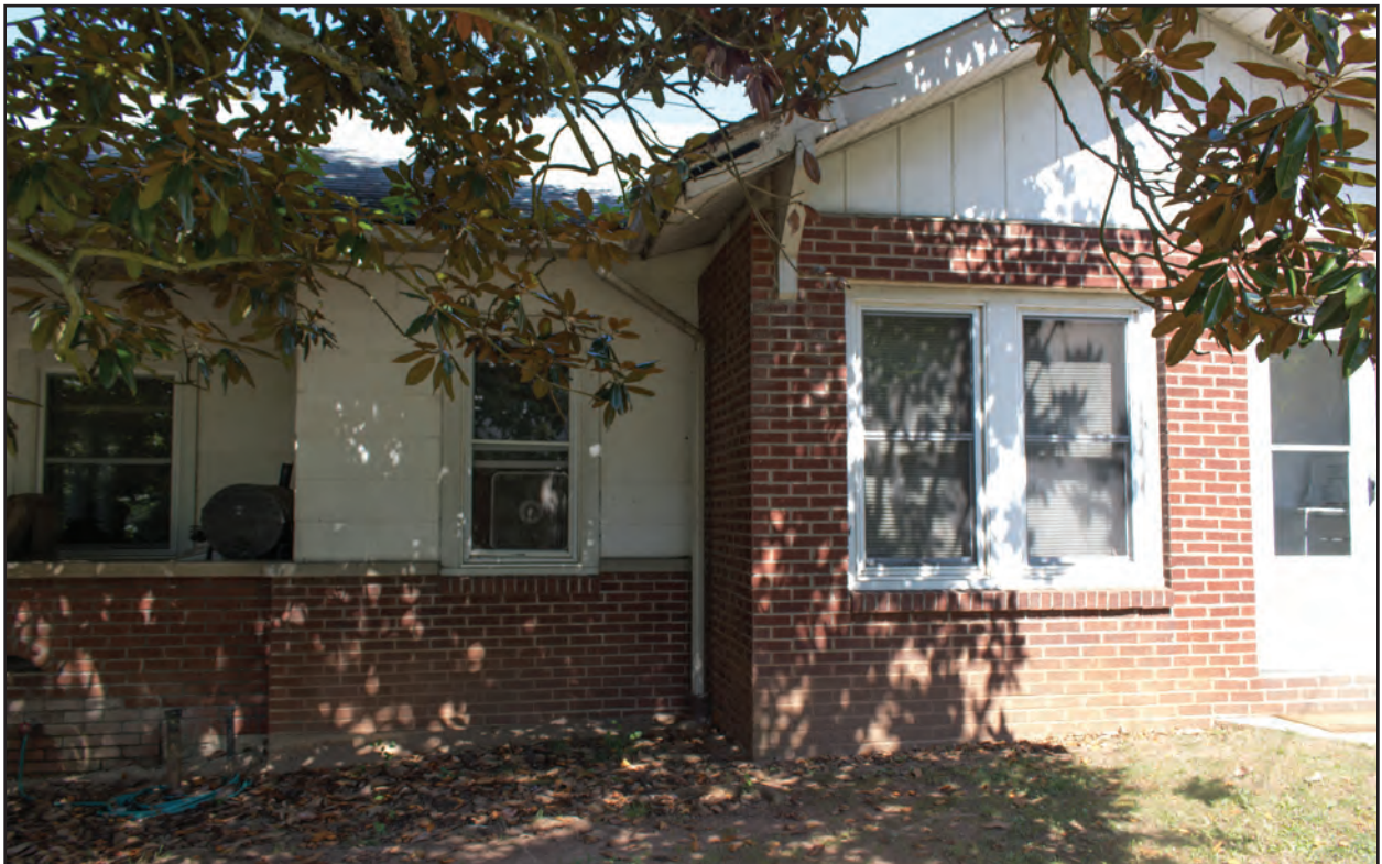
Figure 4.5. 1 Holtzclaw Street, East Side
