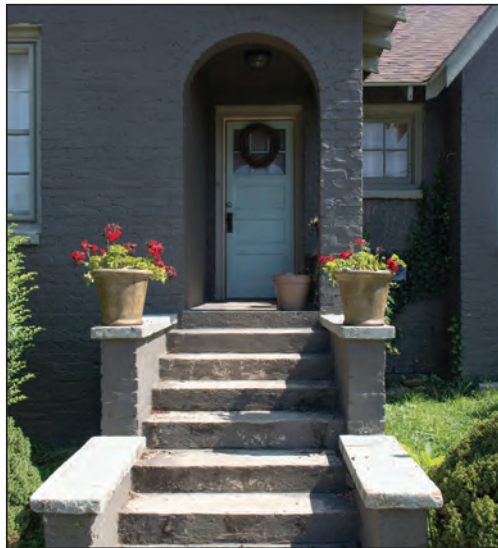
Figure 5.4. 113 Pisgah Drive, Entrance Detail
