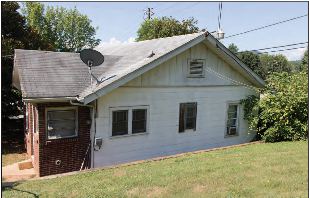
Figure 4.13. 1 Holtzclaw Street, North Side
