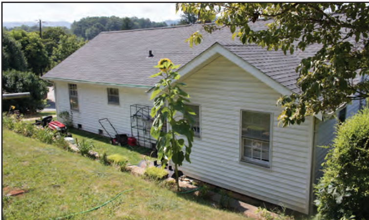
Figure 6.9. 115 Pisgah Drive, North Side
