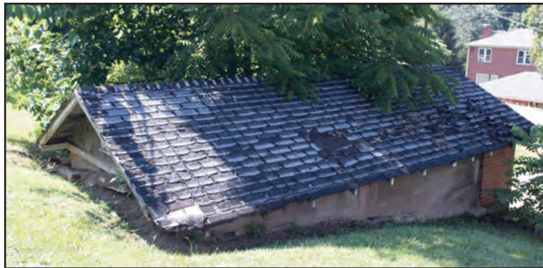
Figure 4.15. 1 Holtzclaw Street, Garage, Roof
