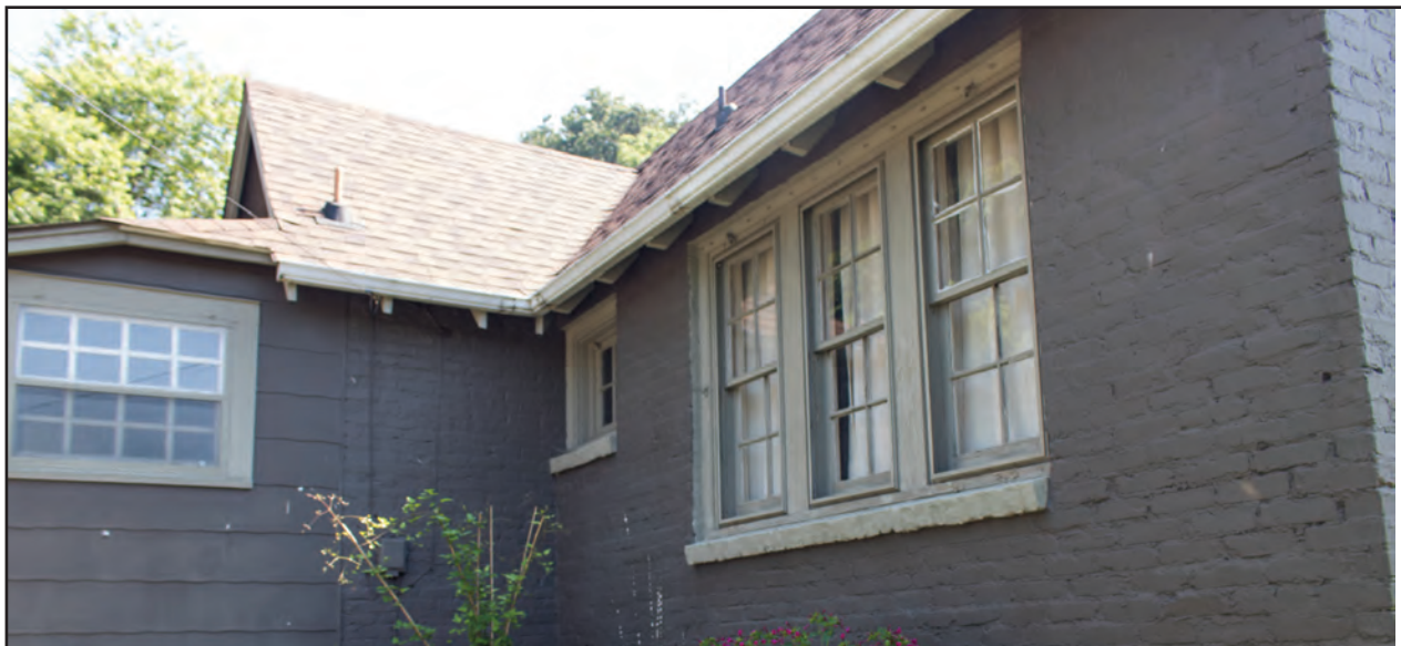
Figure 5.8. 113 Pisgah Drive, West Side, Window Detail
