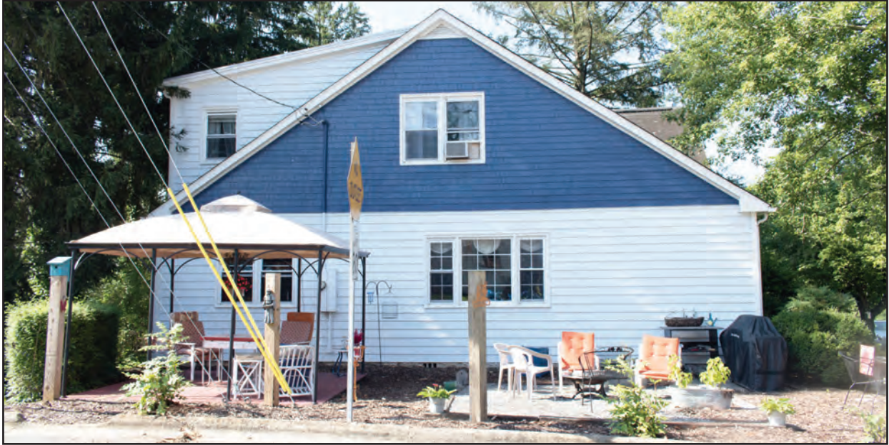
Figure 8.10. 121 Pisgah Drive, North Side
