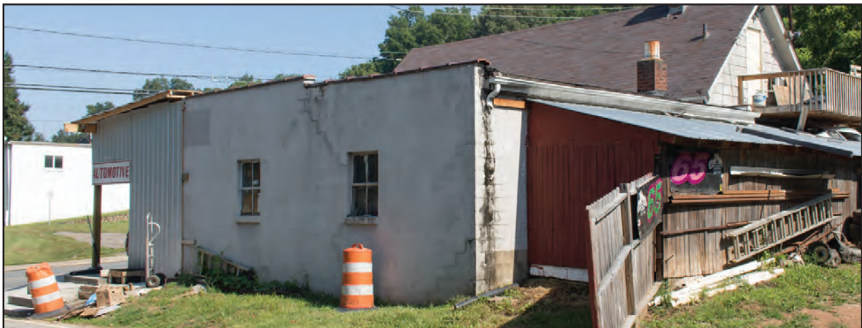
Figure 3.13. Oblique of South and East Sides
