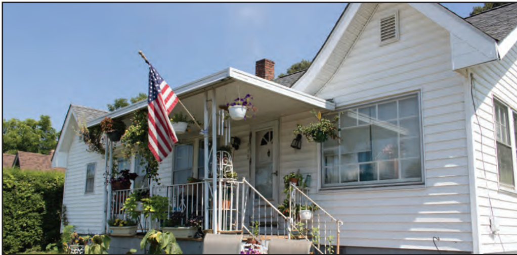
Figure 6.5. 115 Pisgah Drive, Porch Detail, South Side
