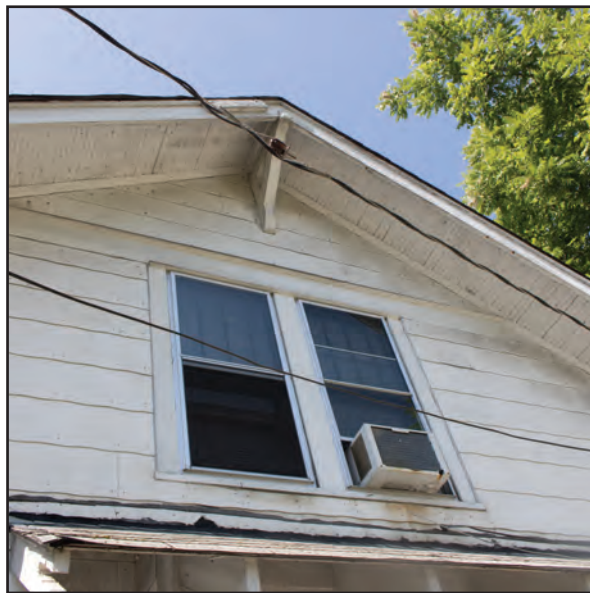
Figure 7.8. North Side, Detail of Upper Floor and Eave
