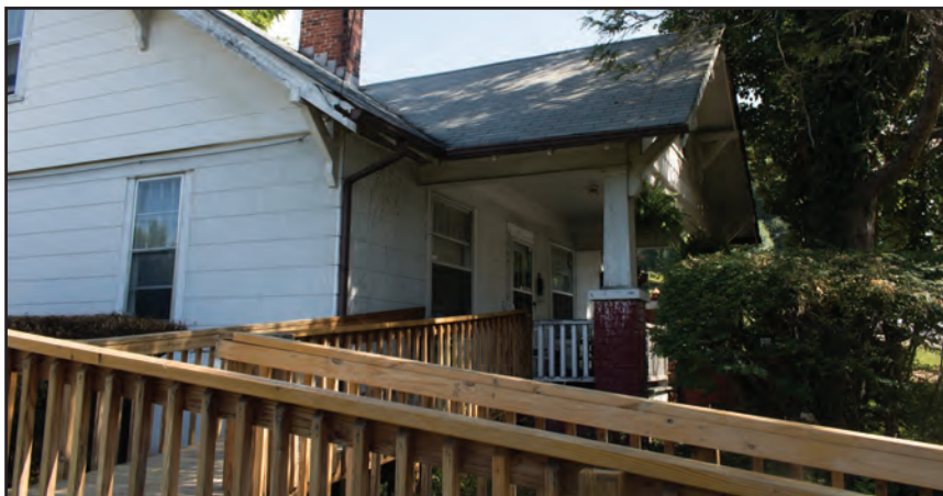
Figure 7.6. 120 Pisgah Drive, View North Toward Porch
