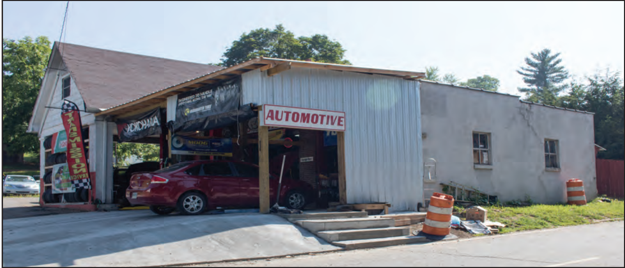
Figure 3.11. Oblique of West and South Sides
