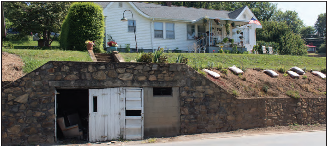
Figure 6.11. 115 Pisgah Drive, Garage on Pisgah Drive
