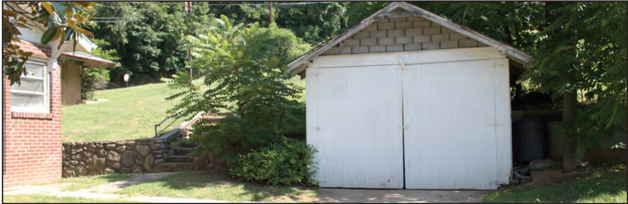
Figure 4.14. 1 Holtzclaw Street, Garage, South Side
