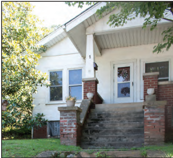
Figure 4.6. 1 Holtzclaw Street, Eave Detail
