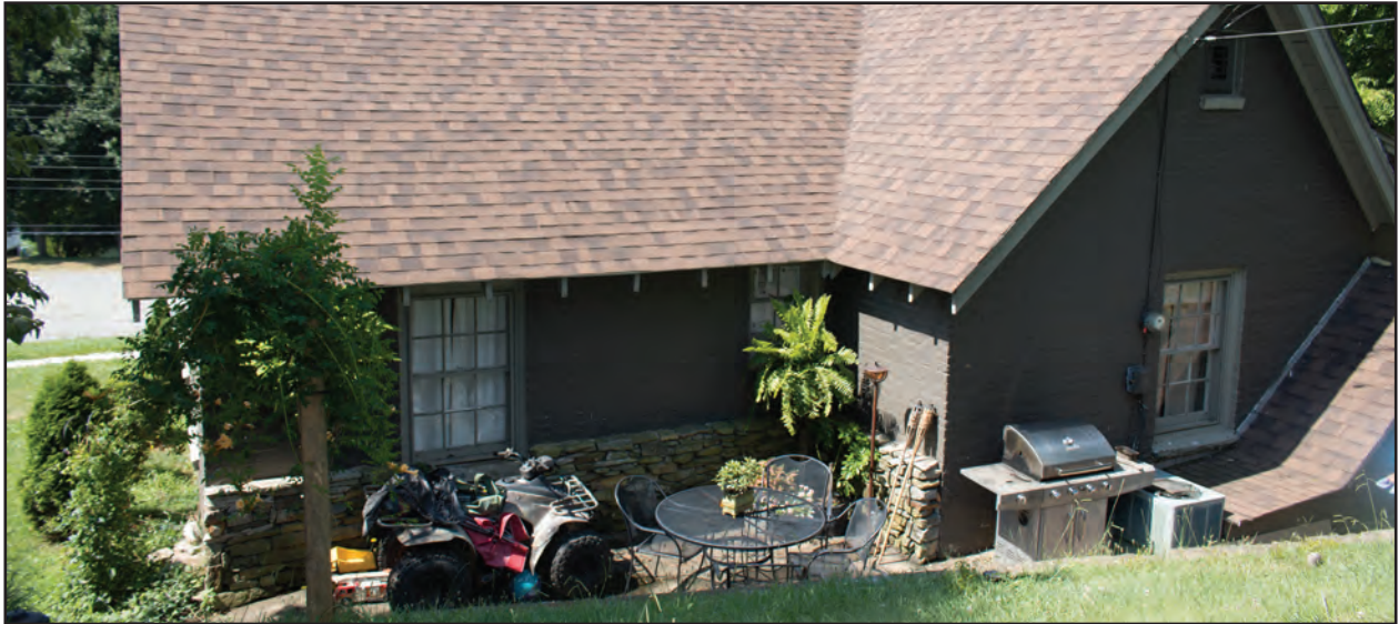
Figure 5.6. 113 Pisgah Drive, North Side
