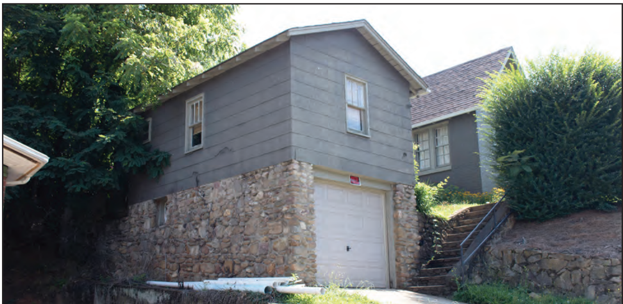
Figure 5.10. Garage, West and South Sides Oblique
