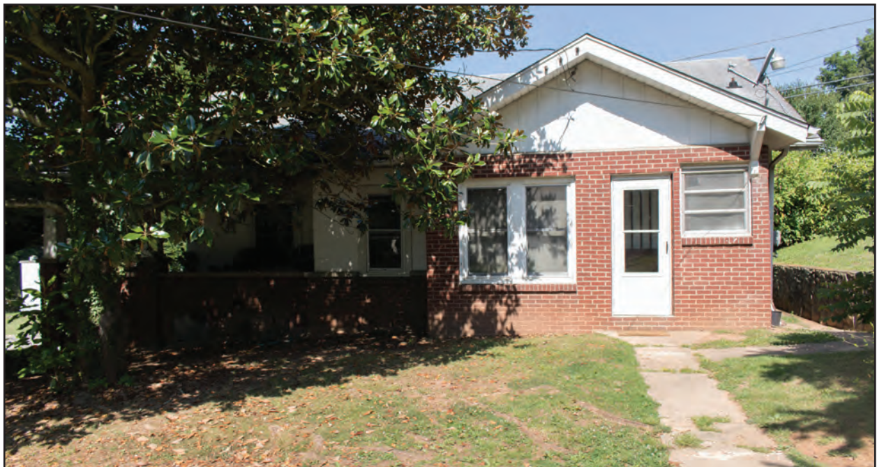
Figure 4.11. 1 Holtzclaw Street, East Side
