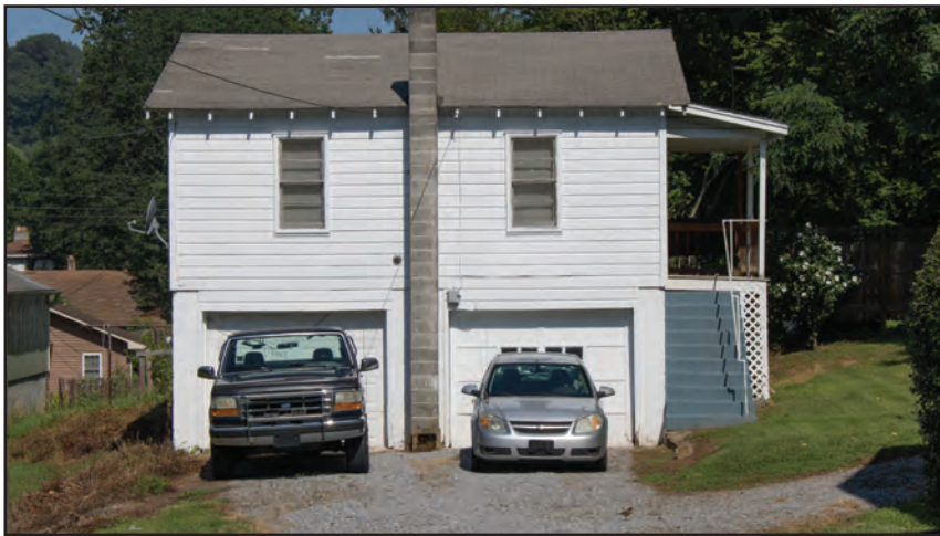
Figure 7.12. 120 Pisgah Drive, Garage
