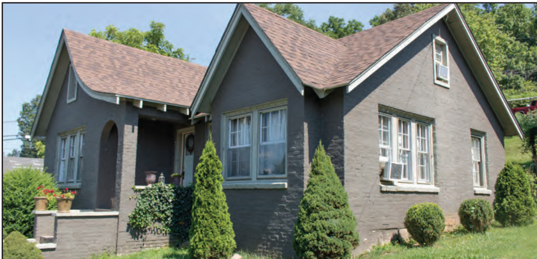
Figure 5.5. 113 Pisgah Drive, South and East Side Oblique
