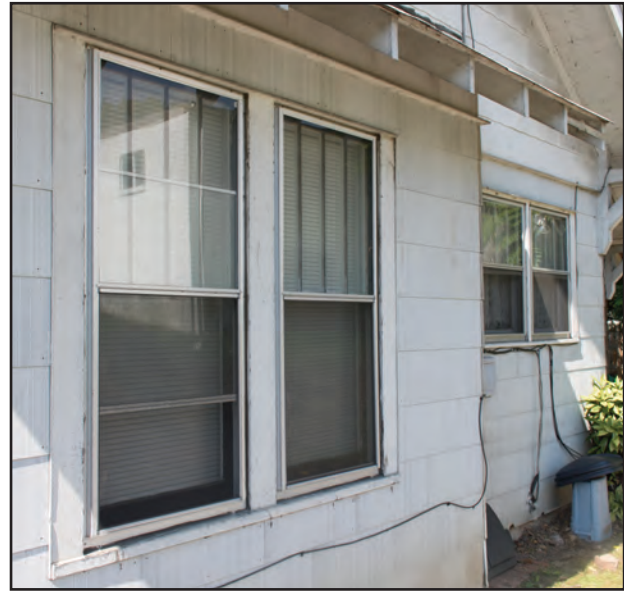
Figure 7.9. 120 Pisgah Drive, North Side, Window Detail
