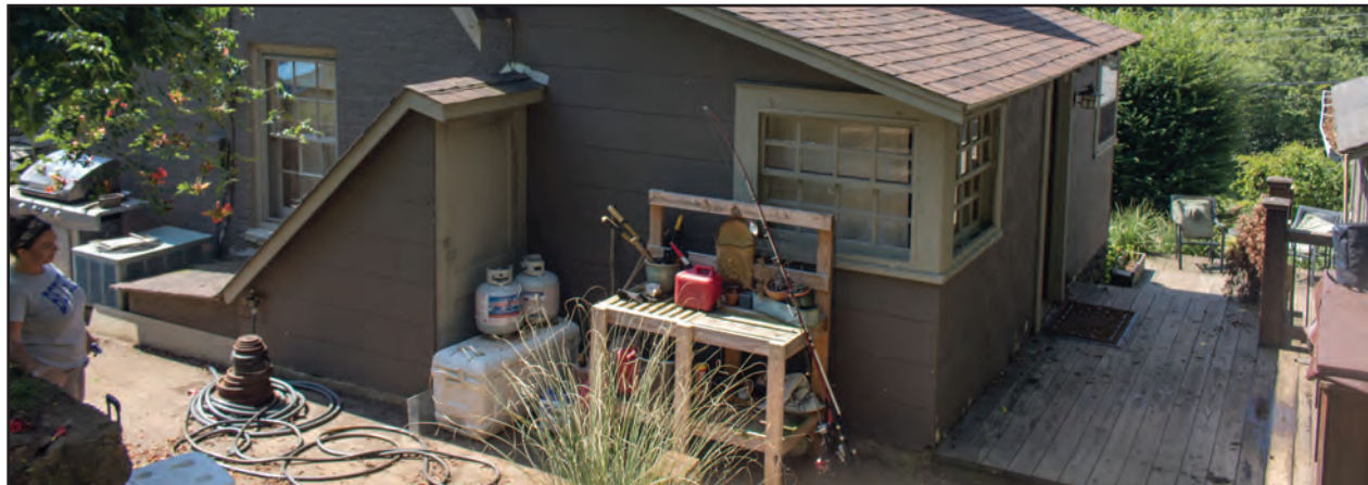
Figure 5.7. North and West Sides Oblique, Rear Addition
